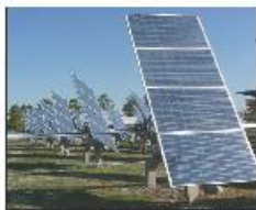
La station de Narbonne
